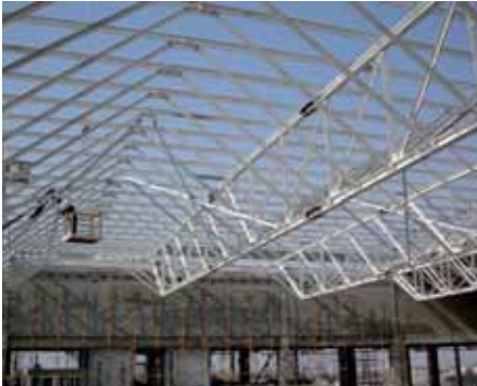
Cairo Airport Terminal Extension, Egypt
